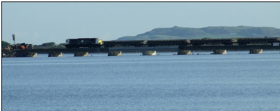
Site 12 – AHC023: Malahide Railway Viaduct, Malahide.
