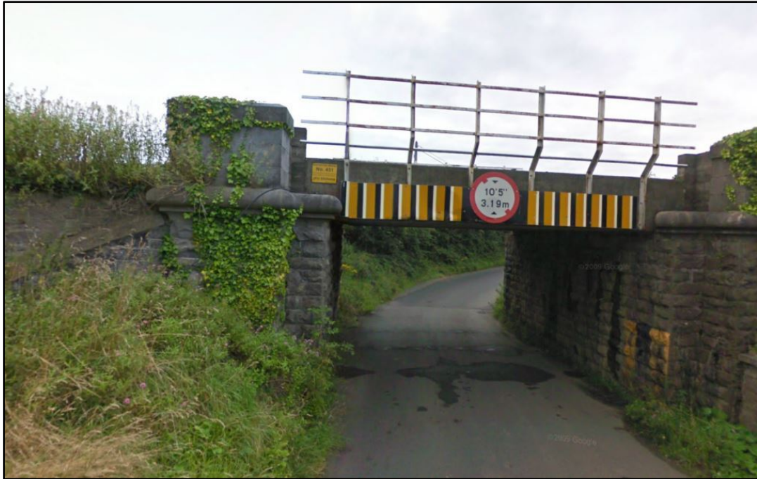
Site 13 – AHC031: Railway Bridge, Kilcrea.
