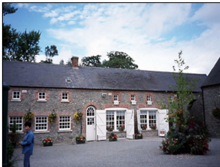
Site 4 – AHC003: Outbuildings, Malahide Demesne.
