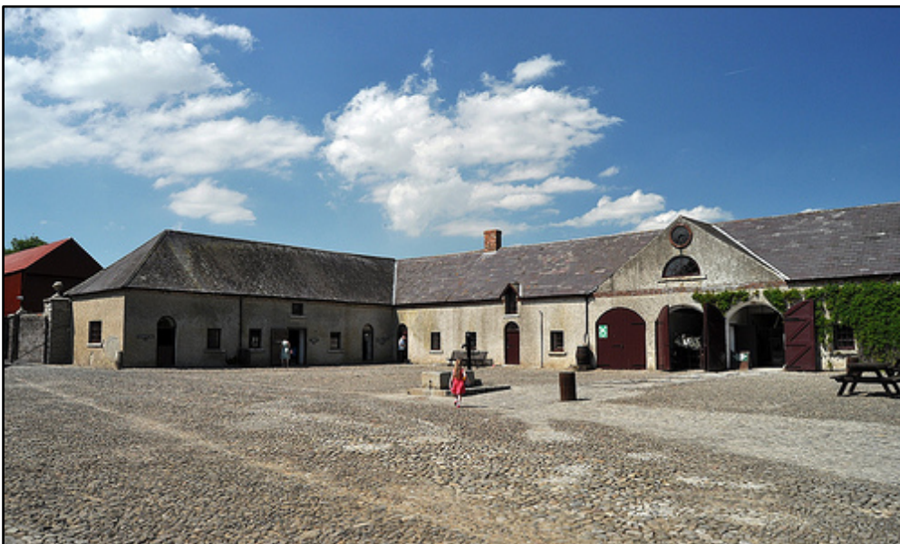
Site 18 – AHC042: Outbuildings, Newbridge Demesne.
