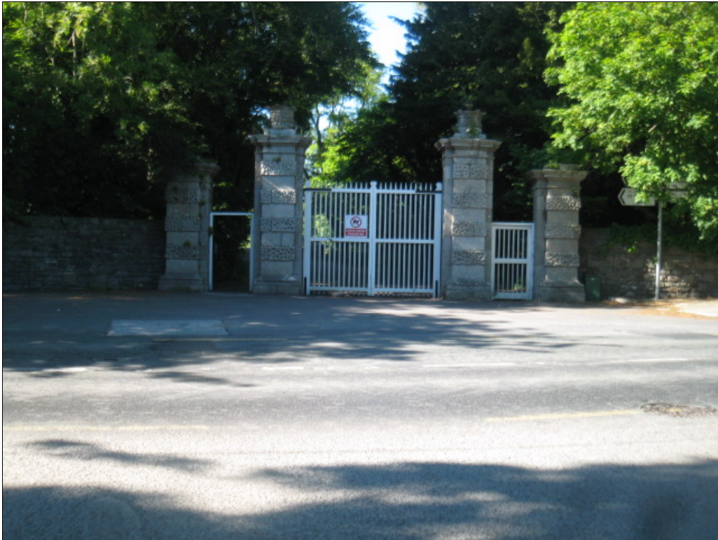
Plate 11: Entrance gates to Newbridge Demesne.
