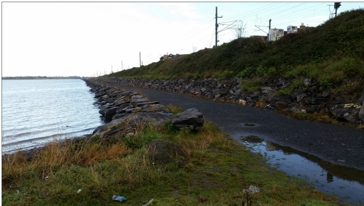
Figure 13 Photo of the existing Weir Maintenance Track
