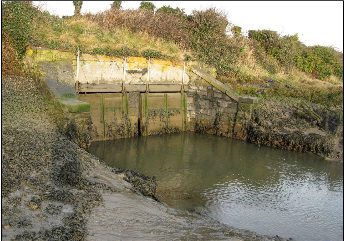
Plate 3: View of the tidal flaps on the River Pill outlet beneath the railway embankment viewed from the Malahide Estuary side.
