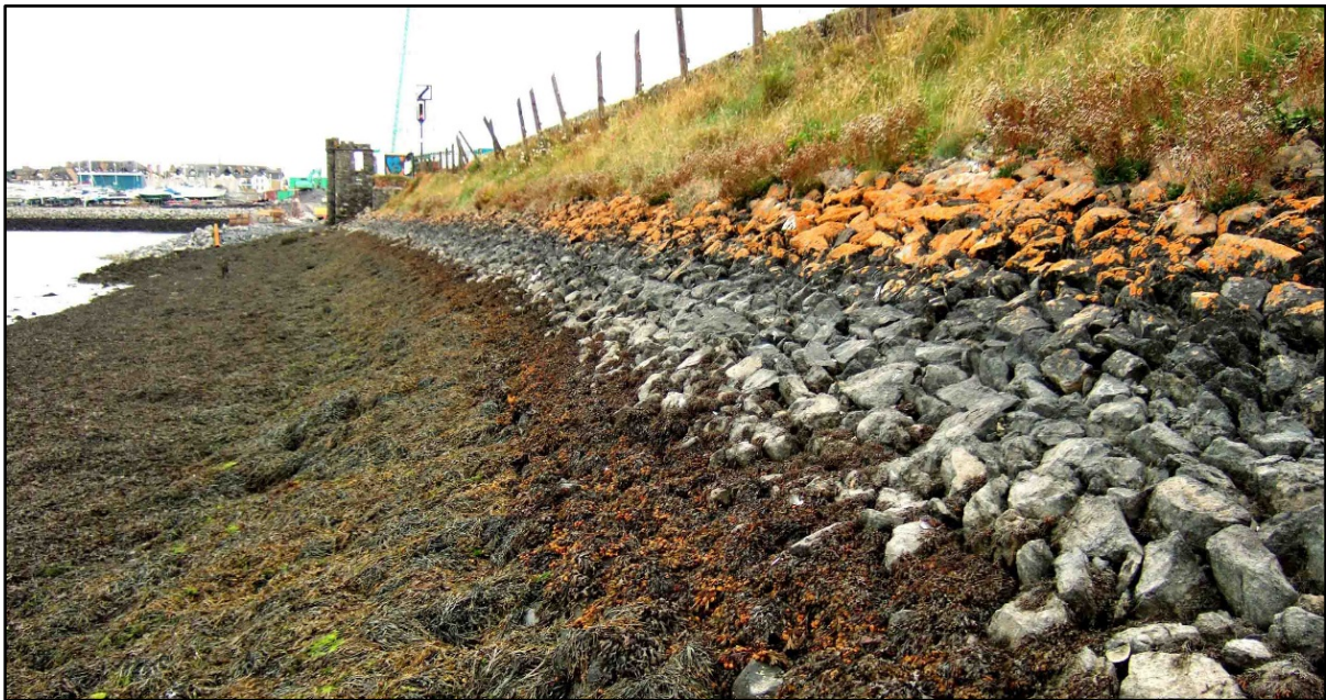
Plate 2: View of distinct vertical zonation pattern along Malahide railway embankment – outer (eastern) face.
