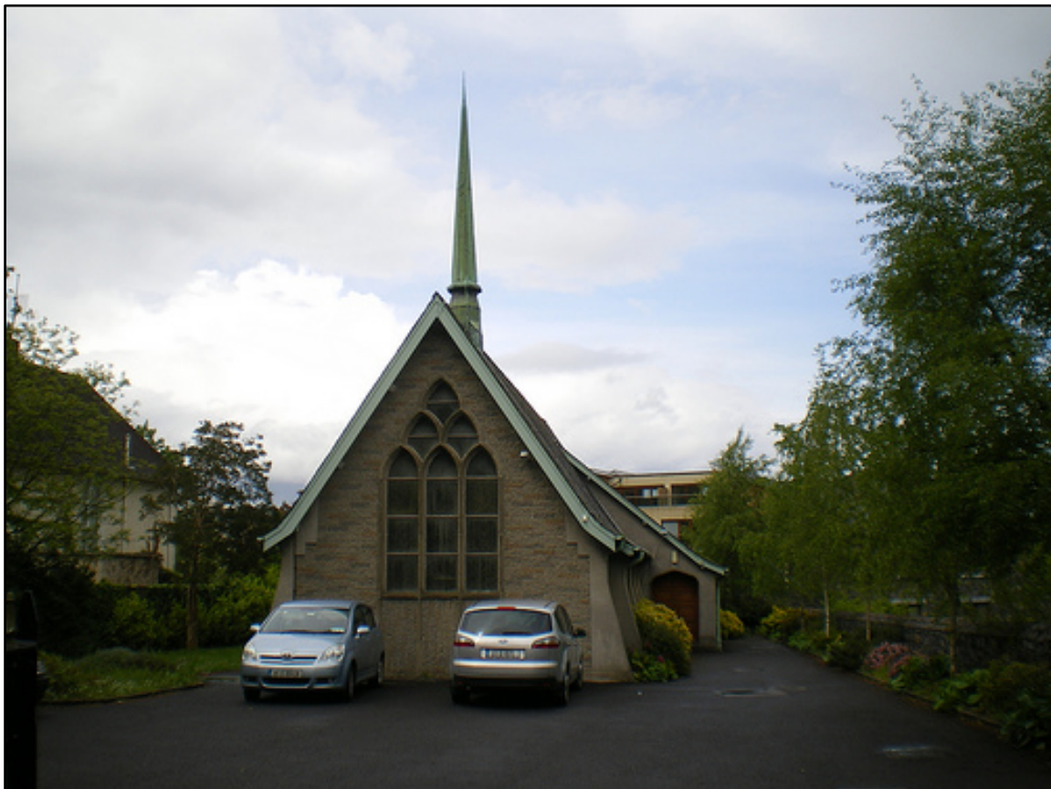
Site 10 – AHC026: Presbyterian Church, Dublin Road, Malahide.
