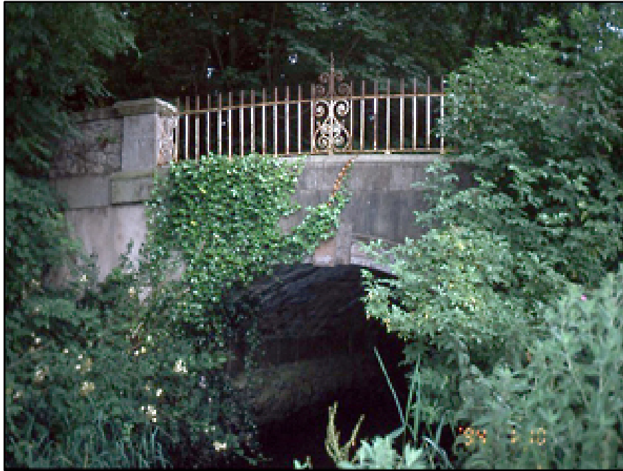
Site 15 – AHC045: Mack's Bridge, Newbridge Demesne.
